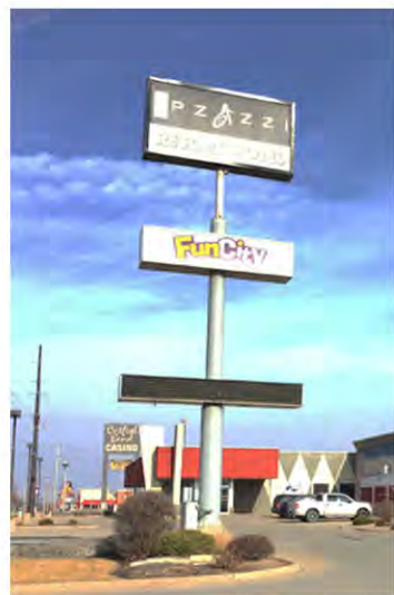
MAIN MARQUEE SIGN - B
